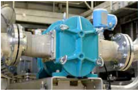
BLUEline pump for conveying cleaning agents
