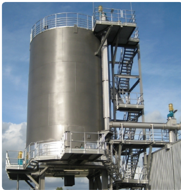
Typical two stage vertical lift sludge conveyors feeding a storage silo
